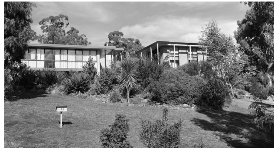
44 and 46 Vasey Crescent, Campbell, designed by Roy Grounds, 1960, in the Melbourne Regional style with long, unbroken rooflines, narrow edge to roof, and glass walls. (Source: NAA, ID Number 11296144)
