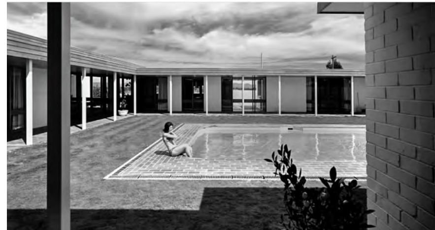
The Birch House, Yarralumla, by Noel Potter of Bunning and Madden, an example of International style in Canberra with low-profile, horizontal form, expanses of glazing and structural crossbeams to create large open plan internal spaces and a courtyard. (Source: Max Dupain and Associates Archives, all rights reserved)
