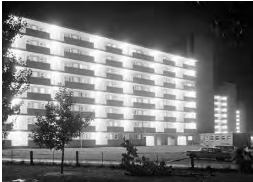
Flats at Braddon at night, 1961. 'The buildings are of reinforced concrete, slanted to get the full benefit of the sun, and flats are fitted with built-in furniture so that tenants need to buy little for themselves'. (Source: NAA, A1200, L37371)
