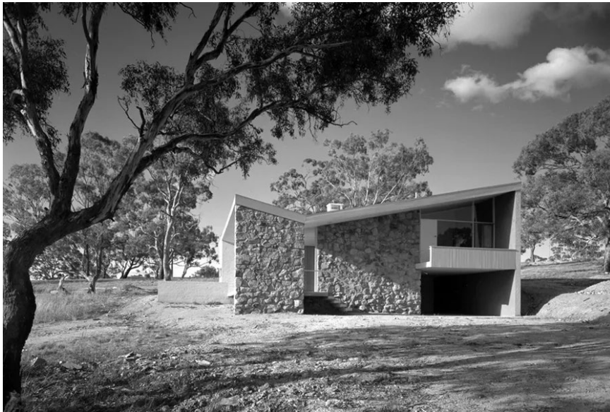
Bowden House by Harry Seidler (1954), a significant International style house in Canberra, with cubiform asymmetrical massing, overhanging eaves for shade, plain smooth wall surfaces, interesting textures and expanses of glass. (Source: Architecture AU, Max Dupain, copyright Penelope Seidler)
