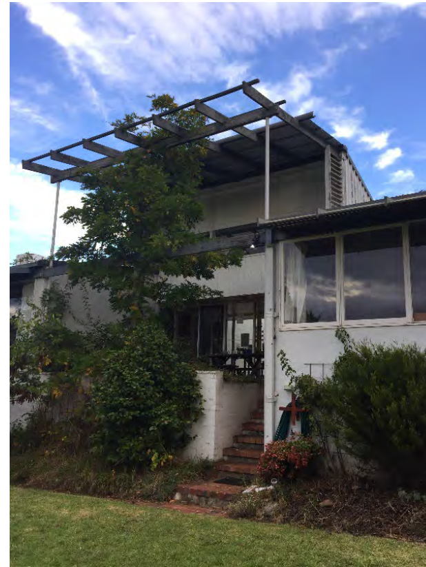
Manning Clark House, 11 Tasmania Circle, Forrest, 1952, designed by Robin Boyd, demonstrates Melbourne Regional style characteristics through the low-pitch gable roof, wide projecting eaves and large areas of timber-framed glazing. (Source: GML Heritage, 2016)
