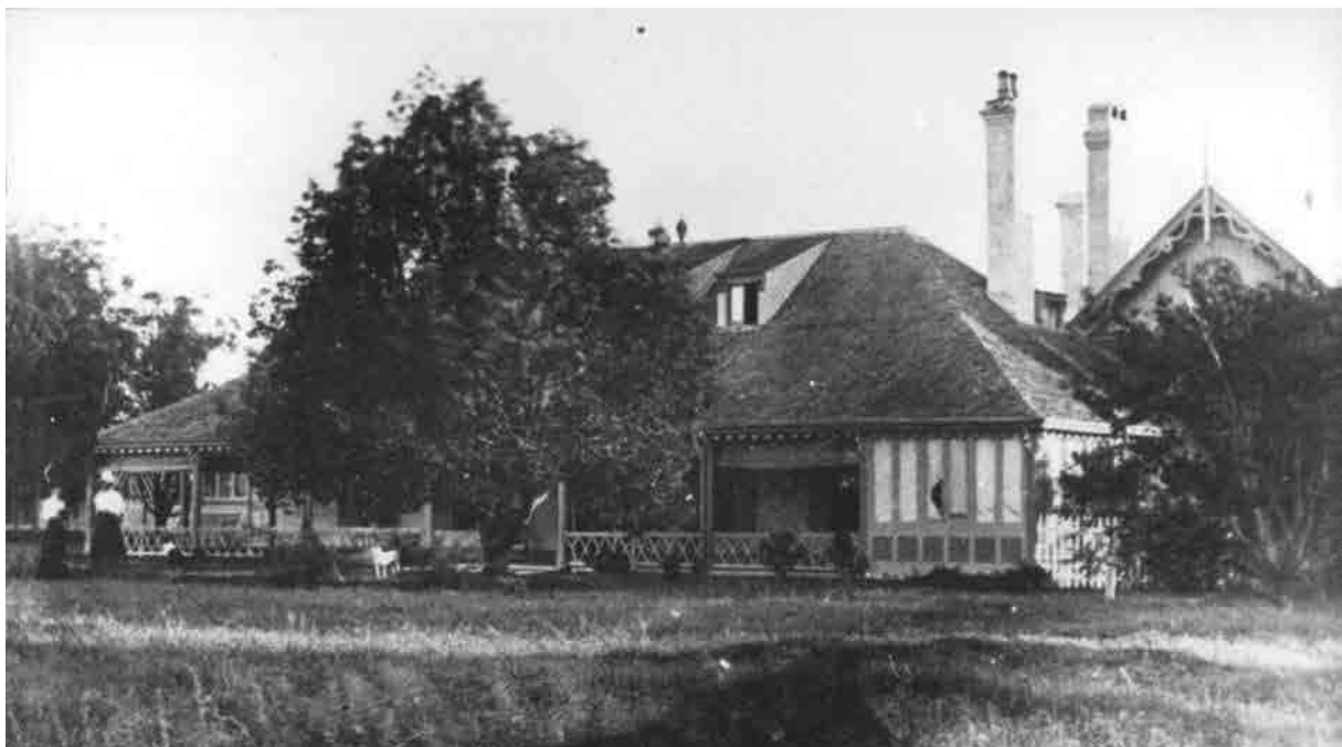
Figure 2.13 ‘Lloydhurst’, the former BNI building, c1906. (Source: Mt Druitt Historical Society)
