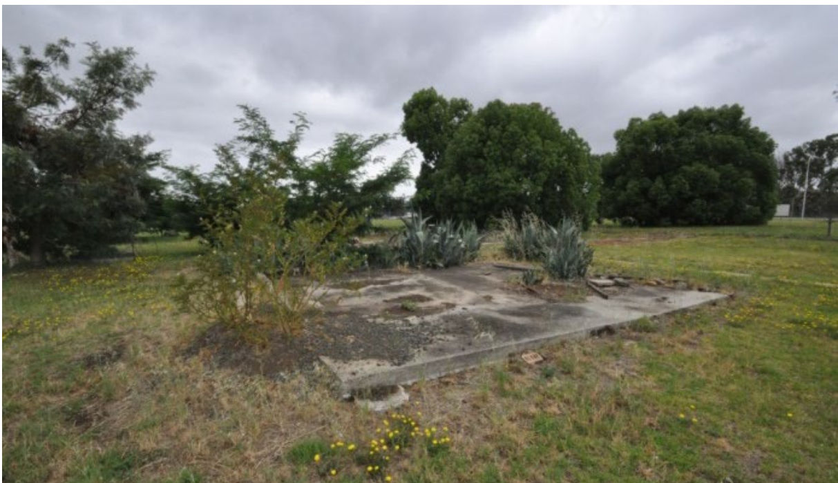
Figure 3.34 A mid-twentieth century concrete slab and remnant garden plantings. Associated with the later cottage. (Source: GML, 2014)
