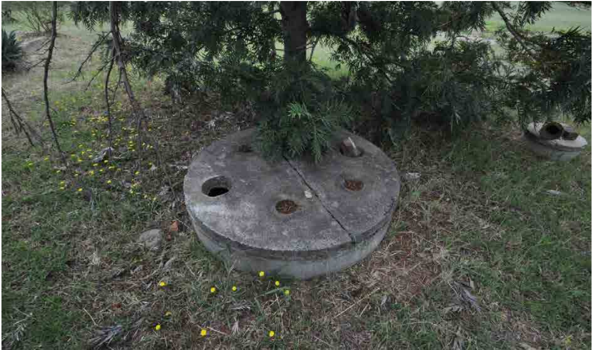
Figure 3.33 Concrete cover over a water cistern. This possibly replaced a former well. (Source: GML 2014)
