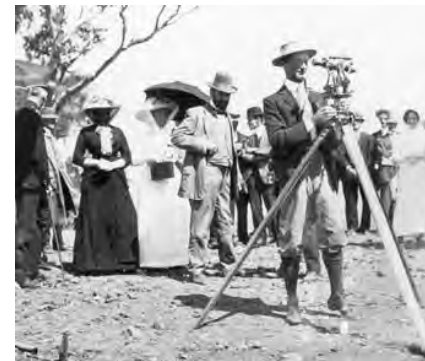
PL Sheaffe, surveyor, determining the second peg on the survey line through Canberra, 1913. (Source: National Archives of Australia [NAA], Item 8357551)
