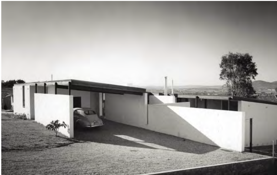
Cater House, 145 Mugga Way, Red Hill, 1965, designed by Sydney School architect Russell Jack of Allen, Jack & Cottier. There is little concern for the façade as a presentation front. Flat roofs, stained timber windows, exposed beams, painted white masonry are all used. (Source: ArchitectureAU https://architectureau.com/articles/cater-house/#img-7 )
