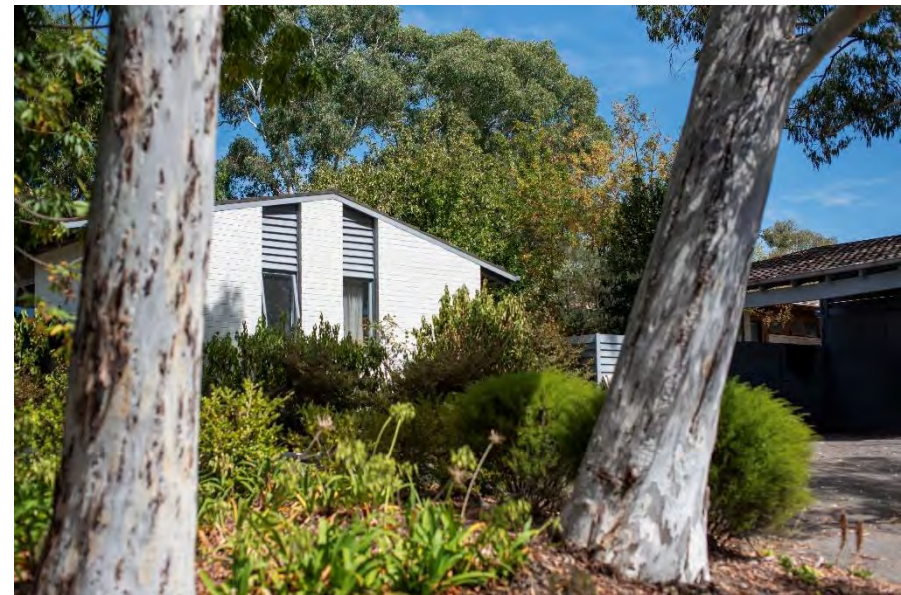
Cameron, Chisholm and Nicol-designed home in Pilbara Place, Fisher, 2024. (Source: GML Heritage)
