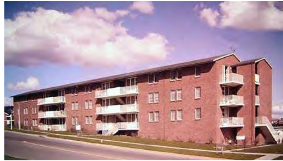
Block of flats at Hughes, 1966. (Source: NAA 1500 K15959)
