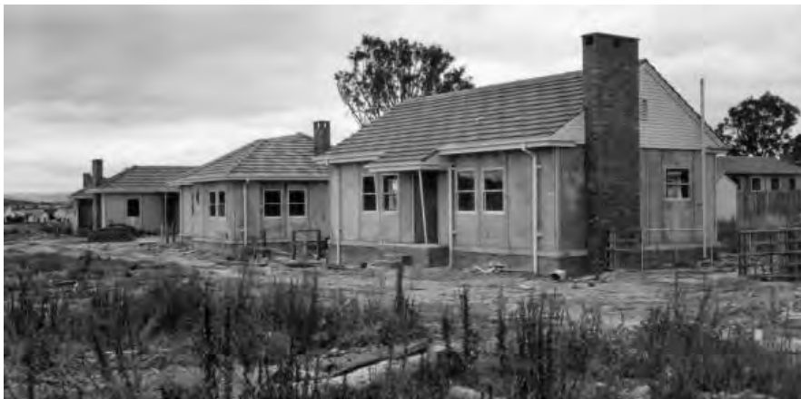
Prefabricated 'monocrete' houses in O'Connor, 1951. (Source: ACT Heritage Library, Ref ID: 001296)
