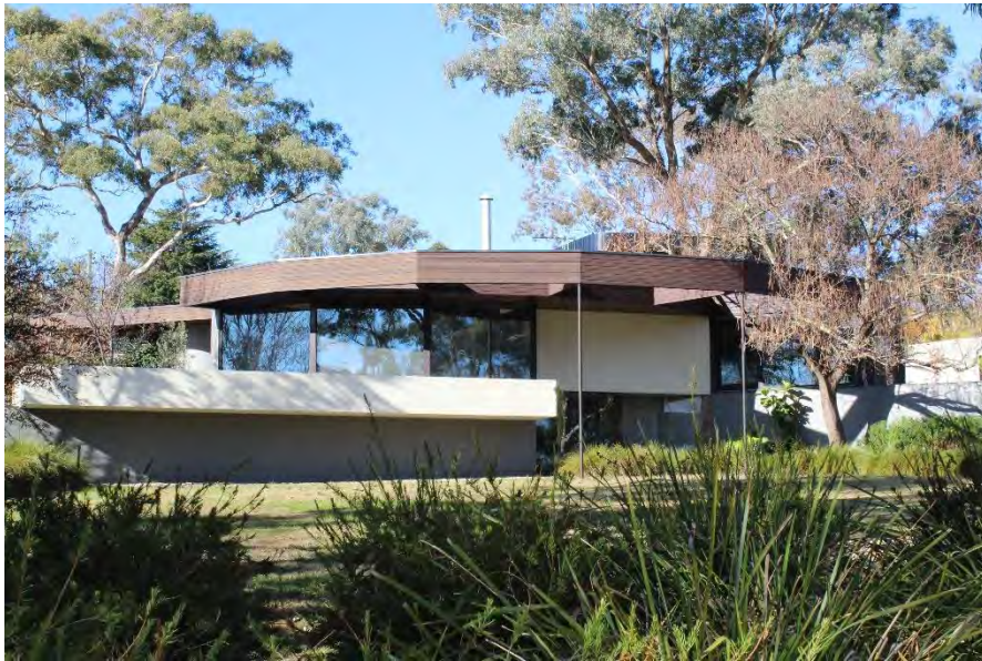
Benjamin House, viewed from northwest. (Source: GML Heritage)
